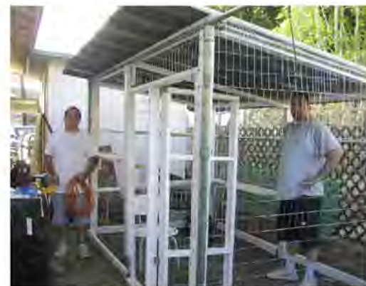
The builders of the Neko House, Paul Marietti and Keith Sato.
